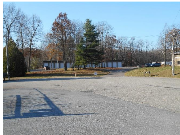
Figure 5: Retrofit proposed in ROW at end of Morse Dr., upslope of Outfall 199.
