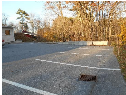
Figure 8: Contois School of Music Parking lot, proposed location of underground infiltration basin.
